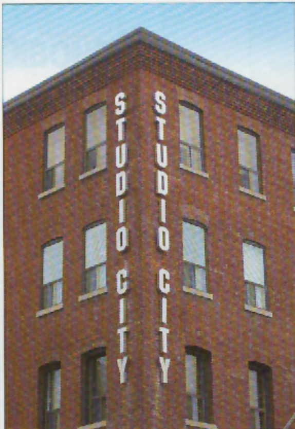
Each of these letters is 3' high. They are aluminum, manually bent with an anodized finish.
