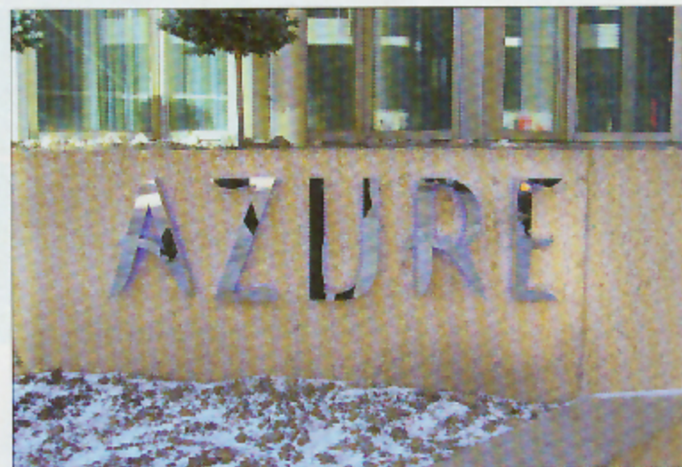
This sign for the Hotel Intercontinental is in the restaurant. They are aluminum letters with a mirror finish sheet that is applied with adhesive. Blue LEDs provide the halo illumination.
