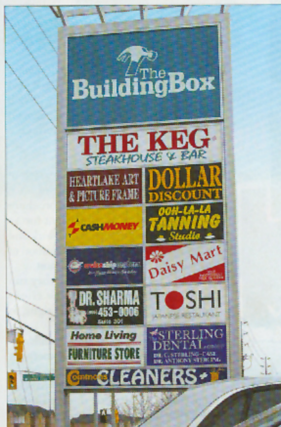
This plaza sign is made up of steel pylon posts, with all aluminum sign frames. All the faces are acrylic with vinyl lettering.
