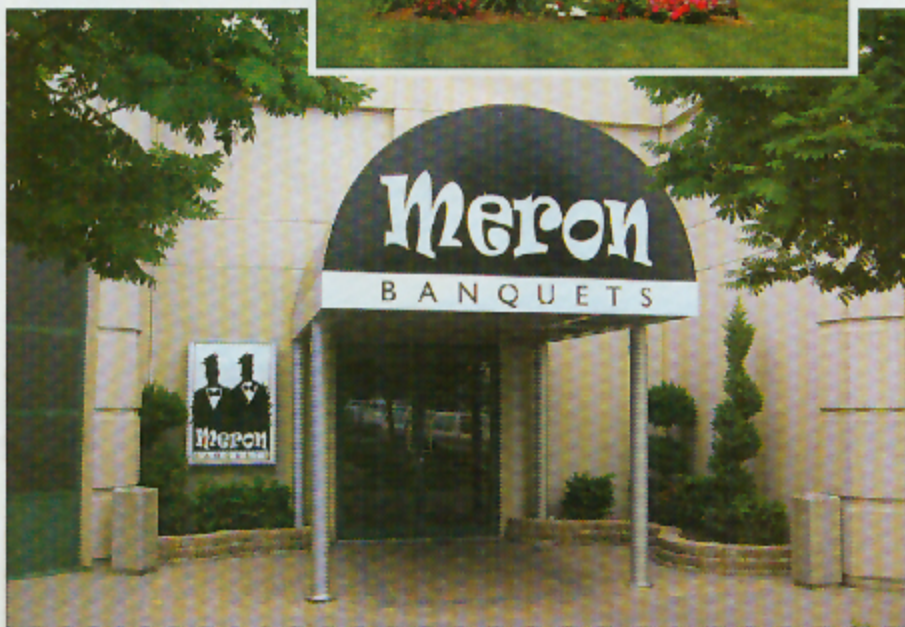
(Below) The lettering was eradicated into the flexible-face awning material for the upper part of this canopy. The white frame around the bottom is aluminum with the "BANQUET" copy furnished in vinyl. All the canopy frames are done in-house at Gregory.
